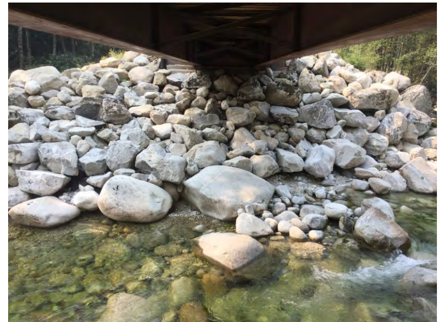
Right Bank Abutment when facing downstream
