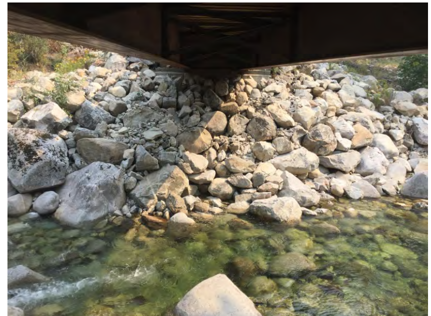
Left Bank Abutment when facing downstream
